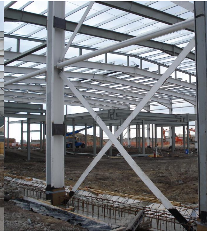
New sports hall steelwork.
