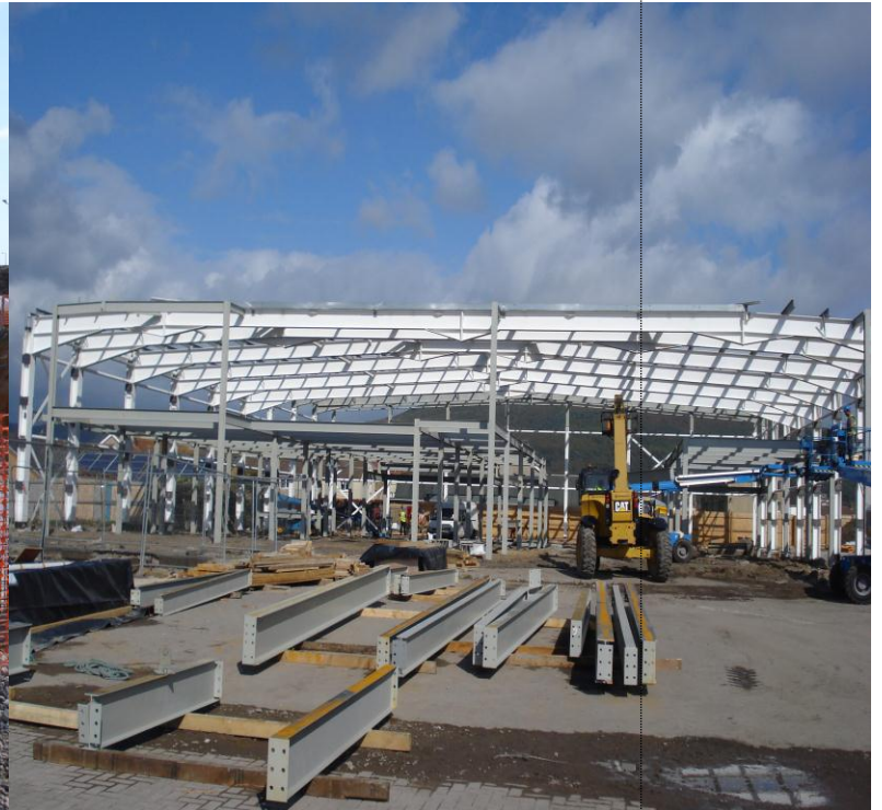
Phase 2 area awaiting steel.
