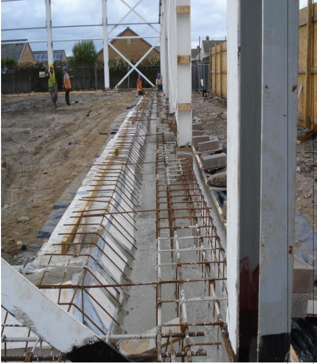
New slab edge detail along GL A.
