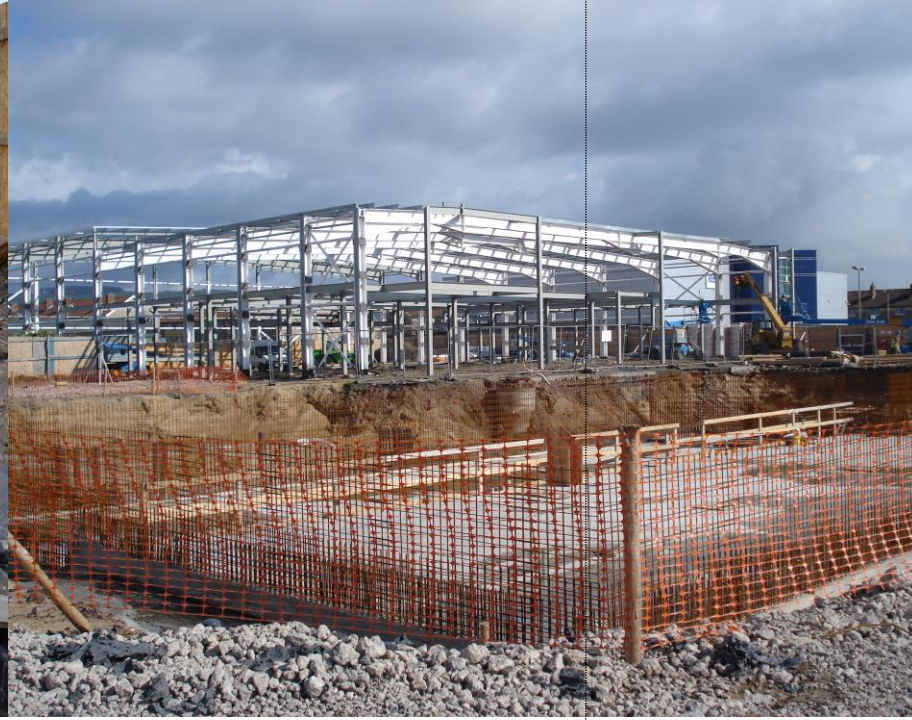
Swimming pool with wall mesh prepared.
